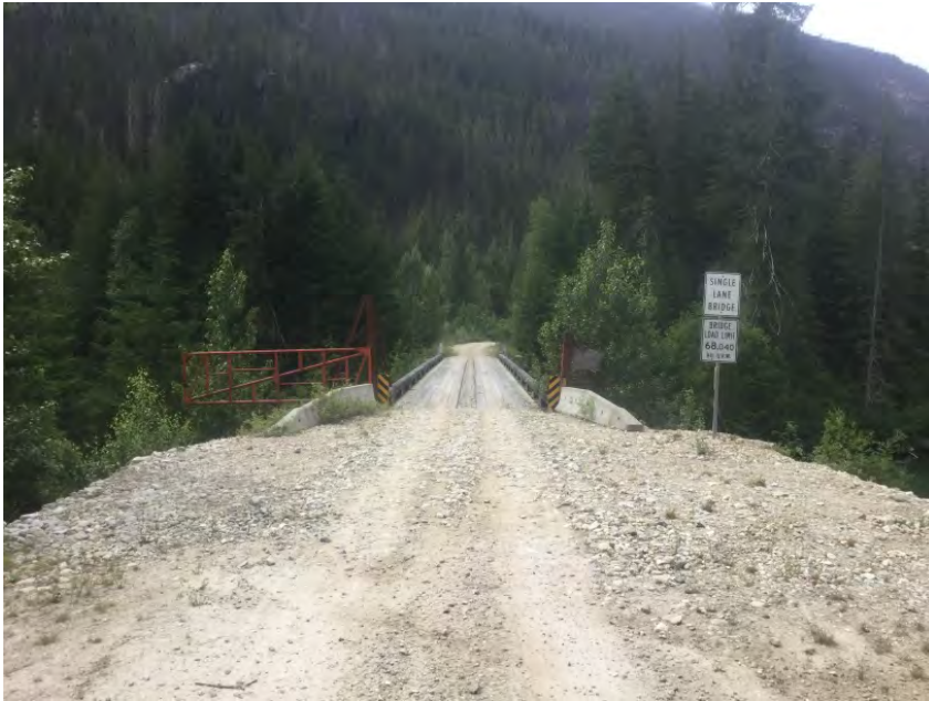
Approach from Left Bank when facing downstream
