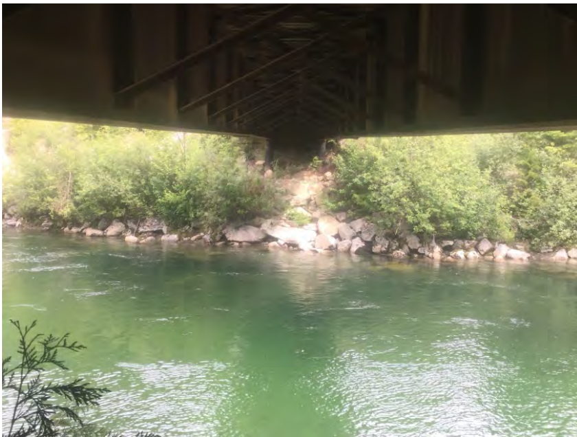
Left Bank Abutment when facing downstream
