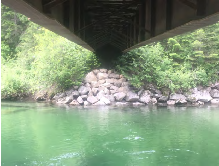
Right Bank Abutment when facing downstream
